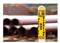
Damage from excavation-related activities is the leading cause of pipeline incidents. To prevent these incidents, we encourage the public to call 811 to have pipelines and other utilities <u>marked before digging</u>. If your property includes an <u>easement</u> and you plan to build, please notify Chesapeake at least 30 days prior to construction.
